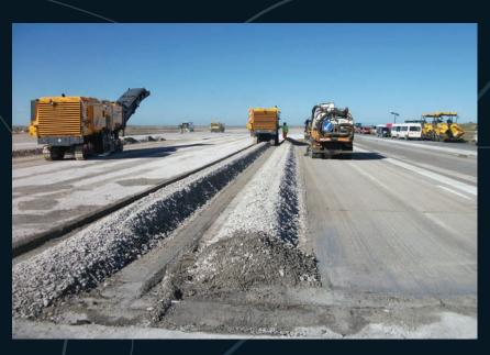
ACHIEVEMENTS: Locally sourced aggregate production – avoiding the import of 30,000 bags of aggregate from an overseas supplier; Aggregate storage plan was produced with consideration of the prevailing winds expected in the Falklands Islands; The re-use of material eliminated any waste and further reduced the quantity of virgin aggregate (bedding sands) that would have been imported from the UK.
